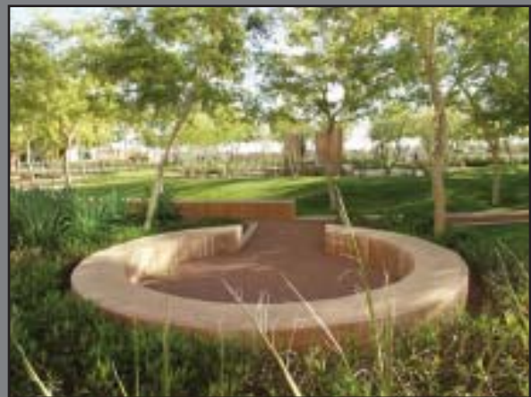
Cast-in-place round concrete bench ringing central green
